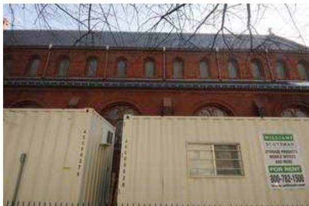
The storage trailers in the 3rd Street Parking
