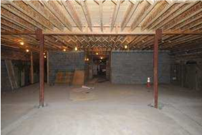
The new undercroft with the new parish hall floor above
