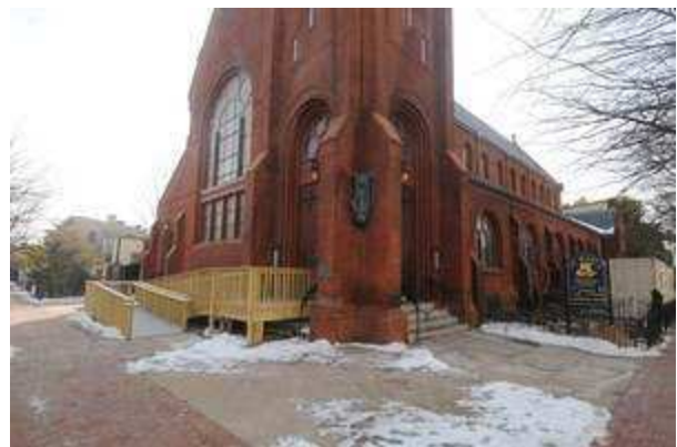
The temporary handicap ramp on the tower corner
